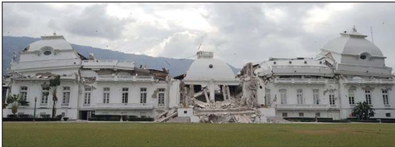
Haiti's Presidential Palace collapsed due to the 7.0 magnitude earthquake that struck Haiti on 12 Jan 2010
