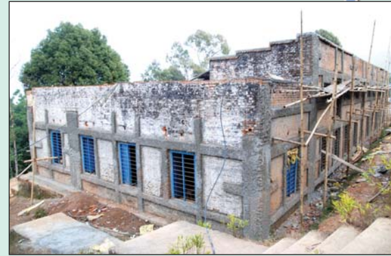
Retrofitting in progress at Shanti Higher Secondary School, Kunchha Lamjung
