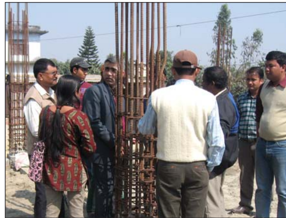
Field visit to building construction site
